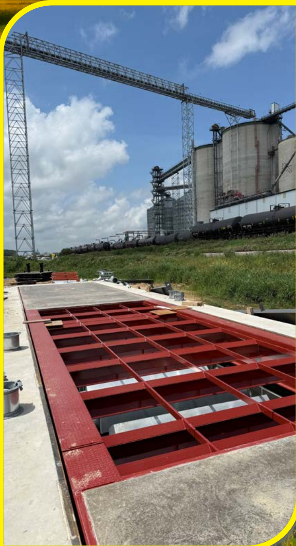
The lane 3 pit is shown here. Once grating is installed, it will be ready to devour your semi load of corn.
